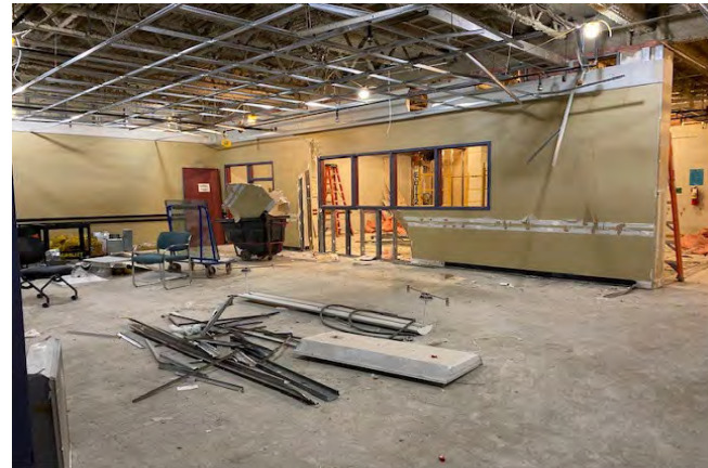
Demolition for Allied Health Simulation Lab
